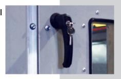
Handles are a thermal bridge issue. Hands can get scraped with door handle. External handle mounted on unit casing.
